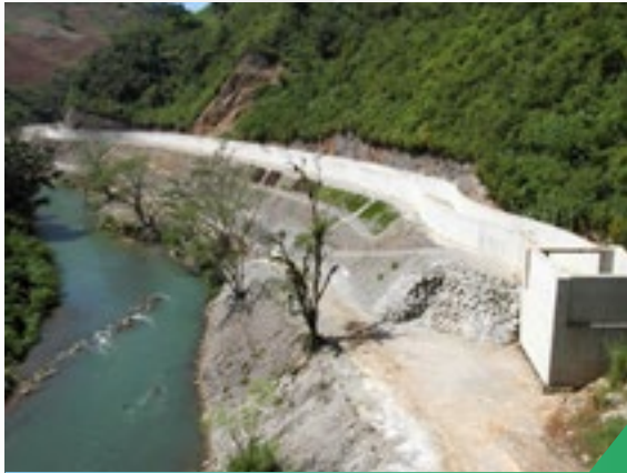
172 Km of Pipelines
